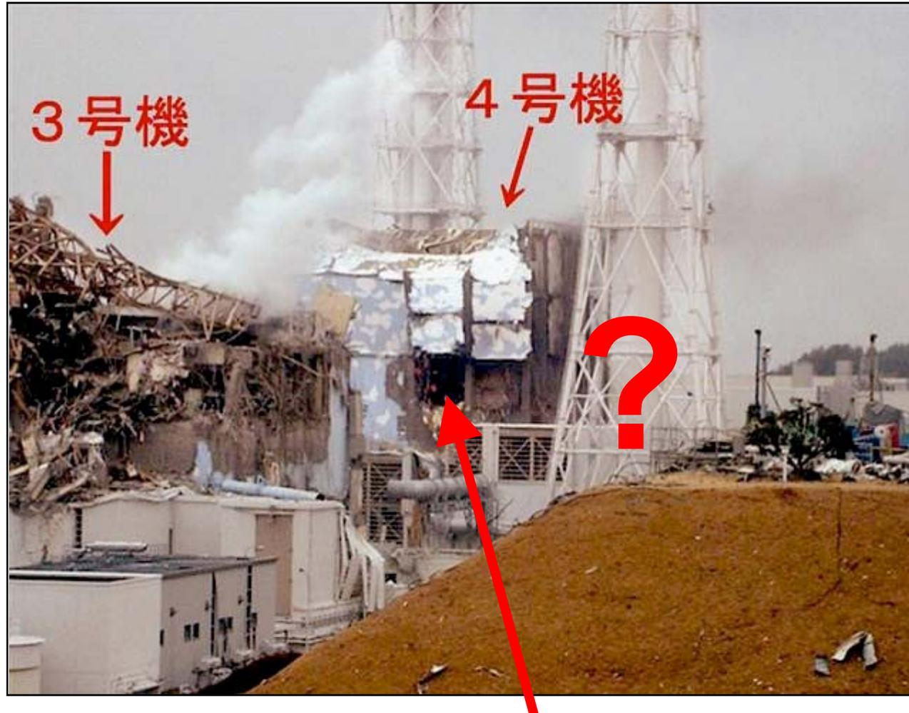
**Explosion in concrete part of the reactor building
