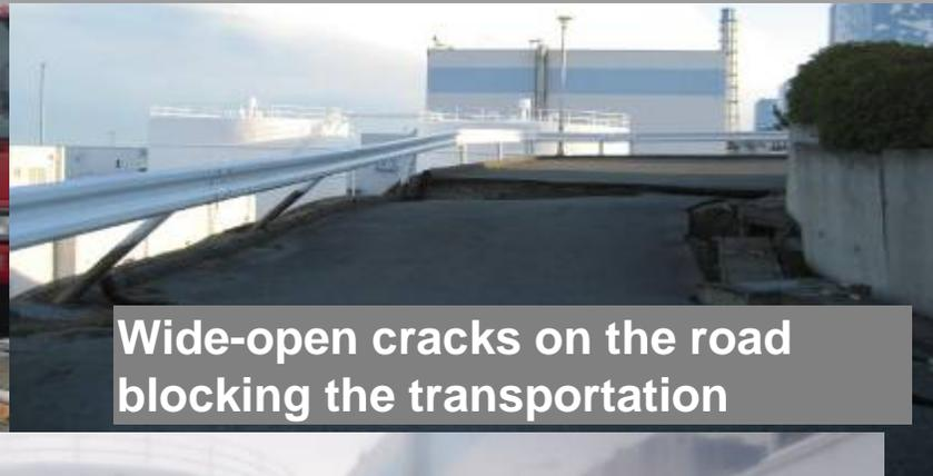
Wide-open cracks on the road blocking the transportation
